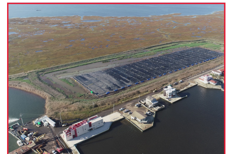
Aerial photo of the DOT's now illegal dredge material facility adjacent to the Edwin B. Forsythe National Wildlife Refuge. Photo attributed to Princeton Hydro
